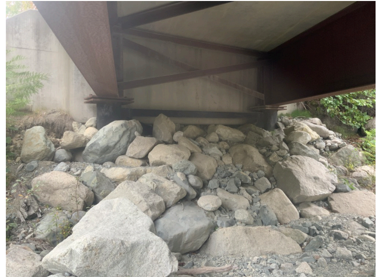
Right Bank Abutment when facing downstream
