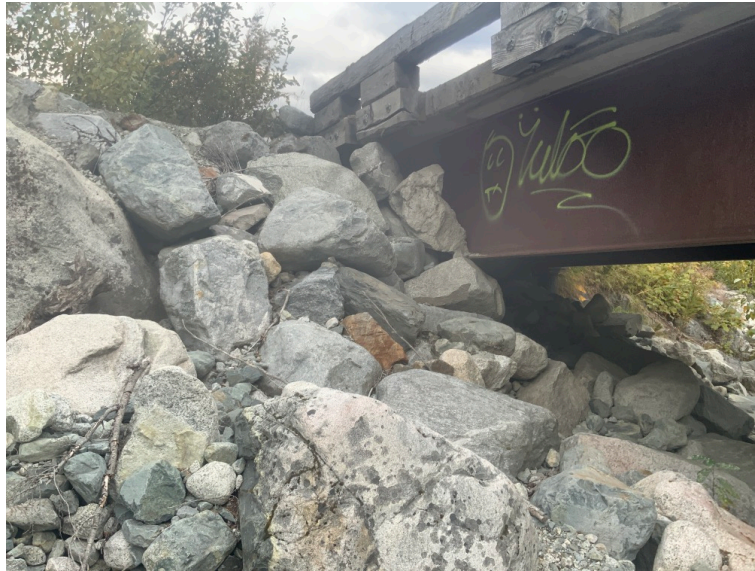
Left Bank Abutment when facing downstream
