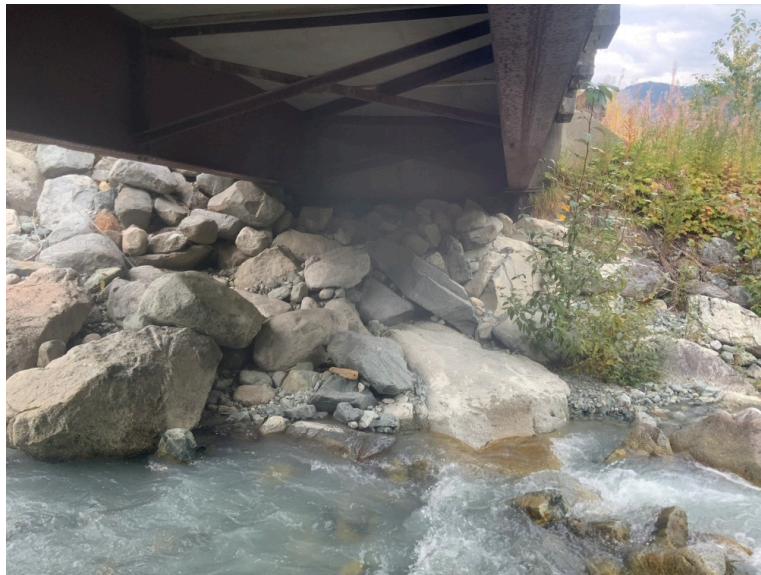
Left Bank Abutment when facing downstream
