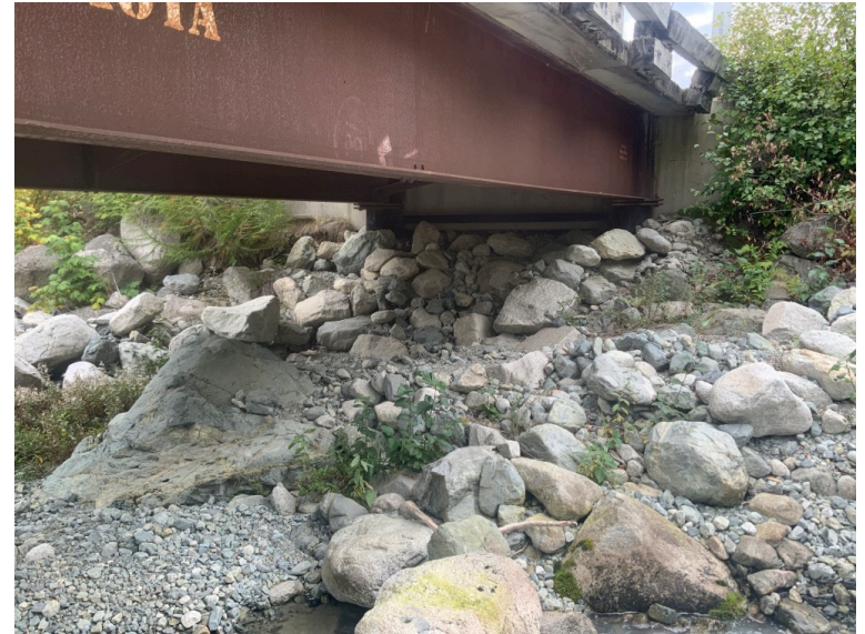
Right Bank Abutment when facing downstream
