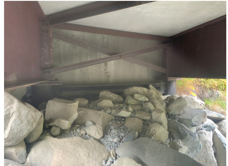
Left Bank Abutment when facing downstream
